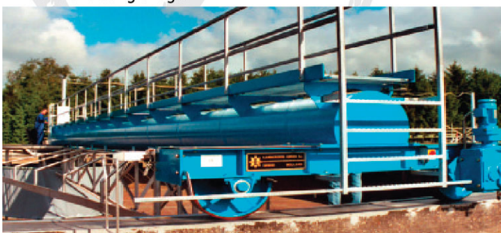
Peripheral driven scraper bridge mechanism with walkway
