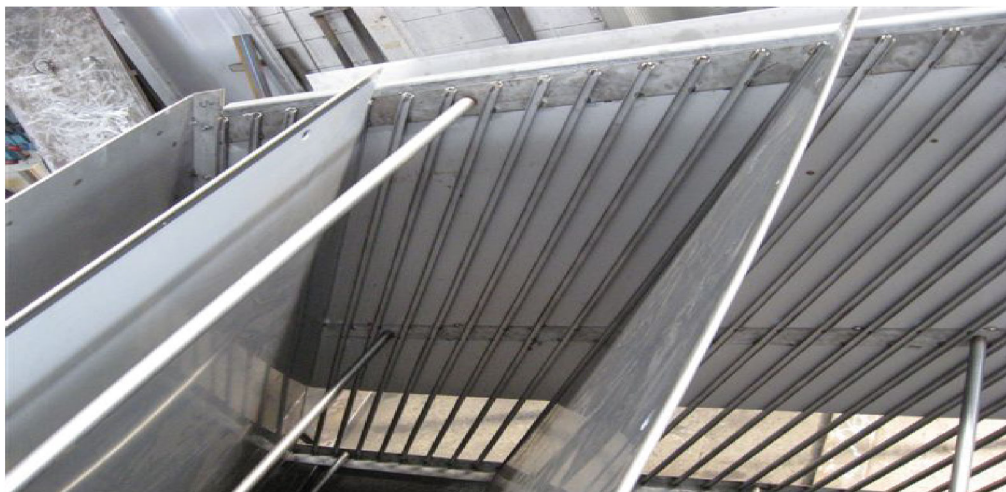
Lamella plate pack frame in AISI-316L during assembly outside clarifier tank
