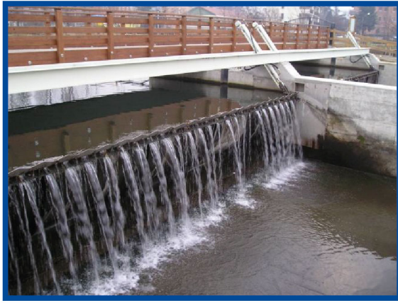
Photo and Sketch of Pivoting Door Weir
