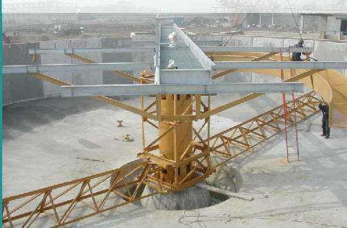
Site assembly of large clarifier scraper
